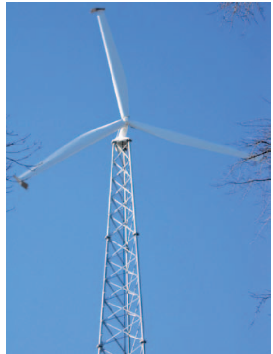
This 50-kW wind turbine is a primary energy source for a municipal office building and water treatment plant in Ocean Gate, New Jersey. Photo credit: Alma Rivera/PIX16904.
