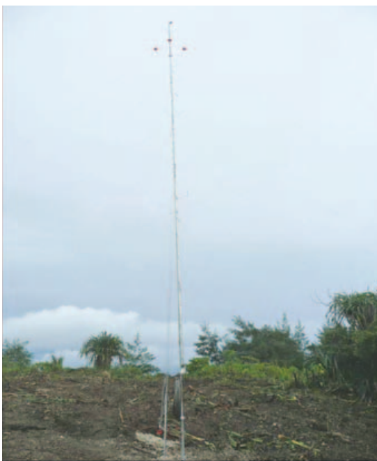
A 60-m anemometer tower on Navy property in Guam. Photo credit: DNV Global Concepts Inc./PIX16289.
