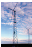
Kotzebue, Alaska Wind Farm consisting of 15 AOC 15/50 or Entegriy EW50 (50 kW); one Vestas V17 (65 kW); and one Northern Power Systems Northwind 100/19 (100-kW).
