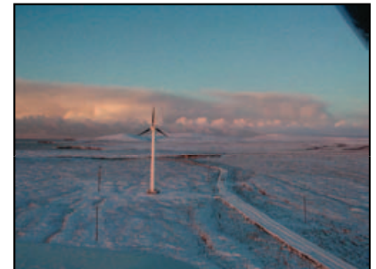
NorthWind 100 turbines in Tuksook Bay, Alaska. Photo credit: Northern Power Systems
