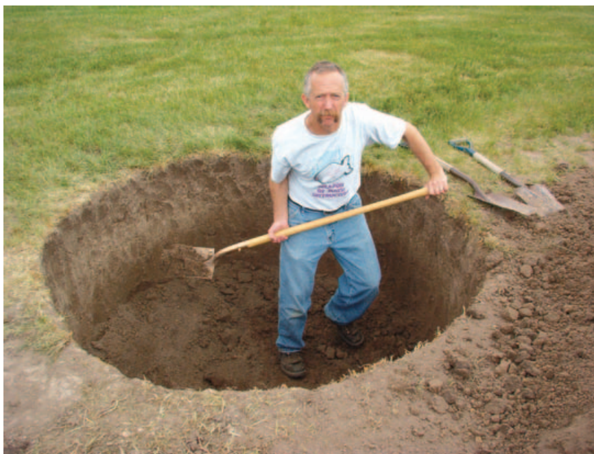
Burlington High School science teacher Jim Jones digs the foundation for the Wind for Schools project turbine. Photo credit: Michael Kostrzewa/PIX16847.
