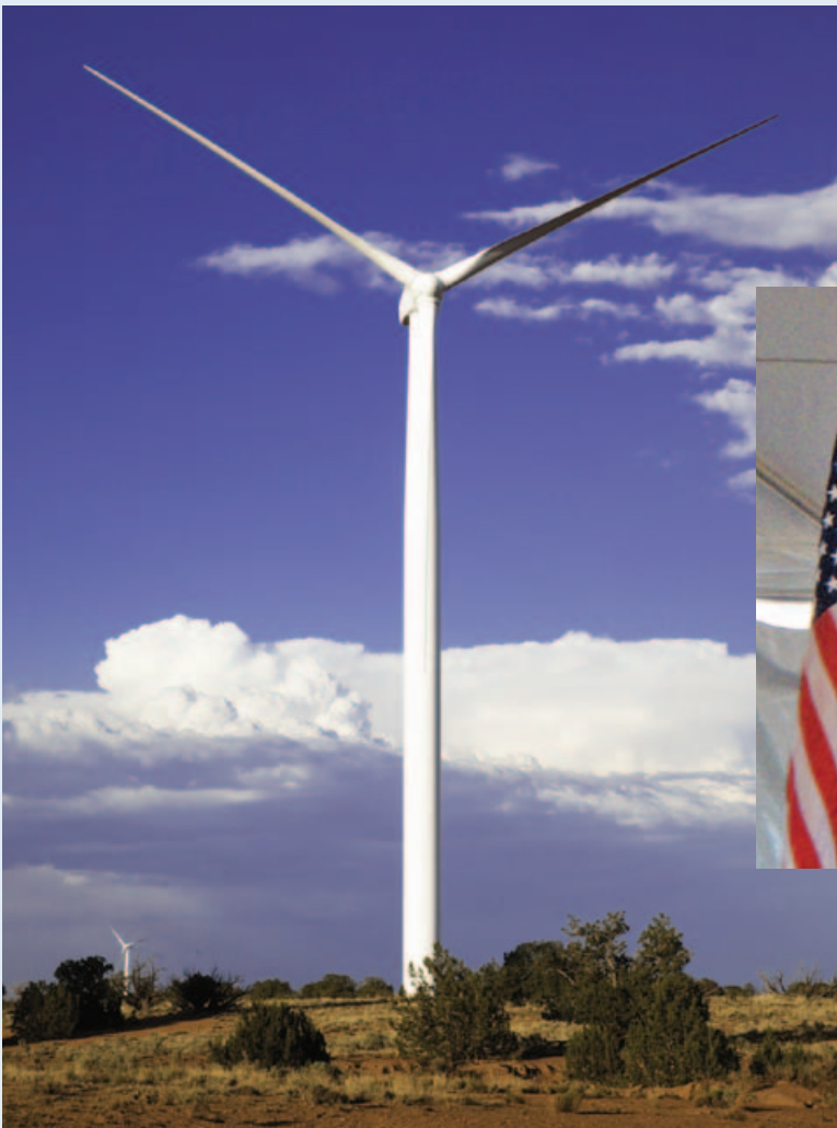
The 63-MW Dry Lake Wind Power Project in Arizona is the state's first utility-scale power project. Photo credit: Iberdrola Renewables/PIX16705.
