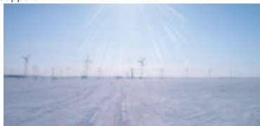
Kotzebue, Alaska Wind Farm consisting of 15 AOC 15/50 or Entegriy EW50 (50 kW); one Vestas V17 (65 kW); and one Northern Power Systems Northwind 100/19 (100-kW).
