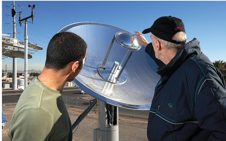
Mechanical engineering professor Bob Boehm, right, and graduate student Ahmad Abu Heiba look at a hybrid lighting system on the roof of Taylor Hall. The dish captures sunlight and transmits it to the building’s interior.
