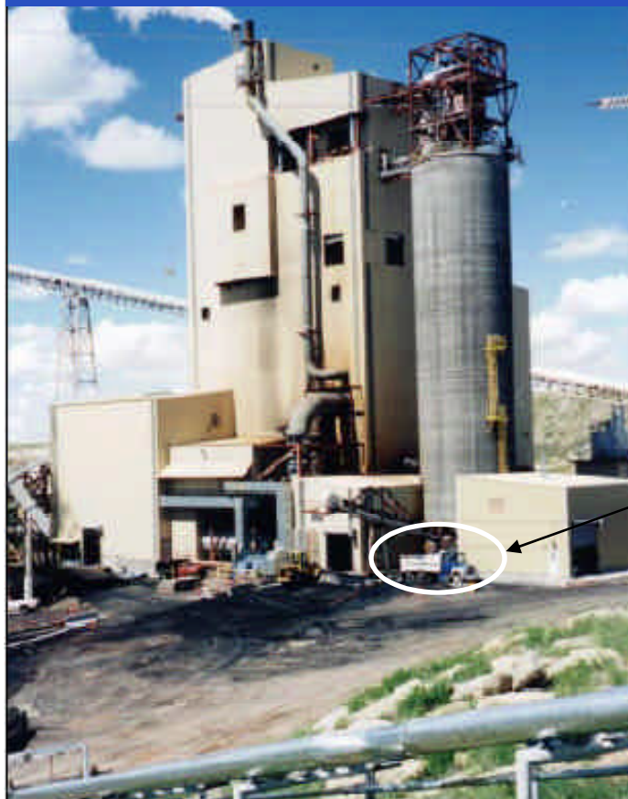
DOE Final Report No. DE-FC21-90MC27339 Sept. 1997 Demonstration plant - 1,000 tons of feed coal per day
