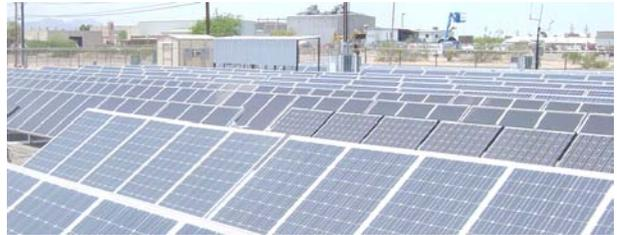
**Figure 1. The TEP solar test yard. Over 600 PV modules from 20 different manufacturers are grid-tied, for a combined 90 kW<sub>peak</sub>. The yard, located at 4350 E. Irvington Rd, Tucson, AZ 95702, was commissioned in 2003. Photo credit: Alex Cronin, NREL PIX 17433.**
