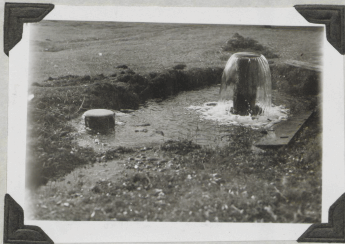
Freak Wells—in Pahrump Valley, same depth, same size casing, eight feet apart. Raycraft Wells #2 and #3.
