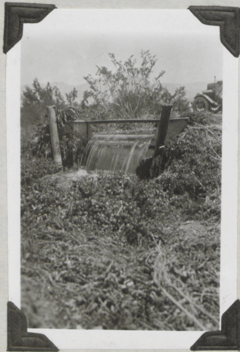
Pump Test of above Well. Yield at 47 feet, 2.23 cfs.
