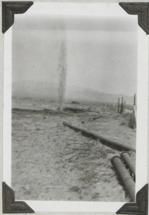
Shooting Boul Well #2, result of a 70# charge of 80% gelatine.
