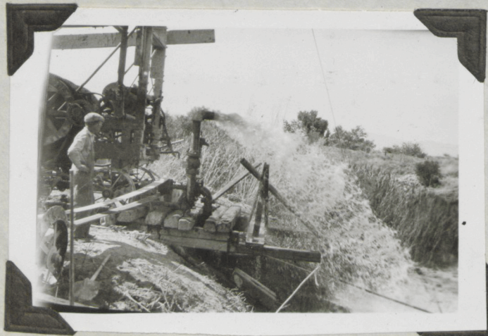
Pumping Taylor Well #4, yield 1.90 cfs, at 23 feet drawdown.
