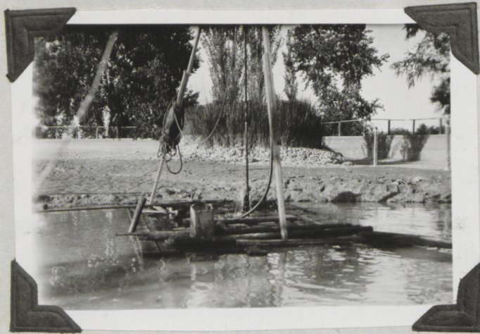
Drillin with hand rig in old spring at Taylor Ranch.
