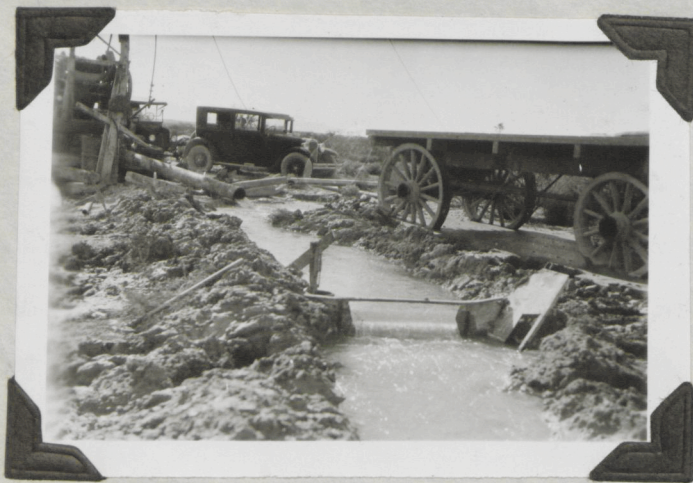
Pumping the Taugher Well yield - 1.50 cfs, at 15 foot drawdown.
