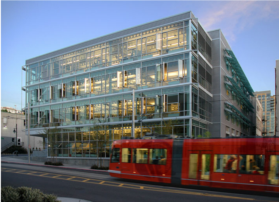
Figure 21.0: Terry Thomas Office Building
