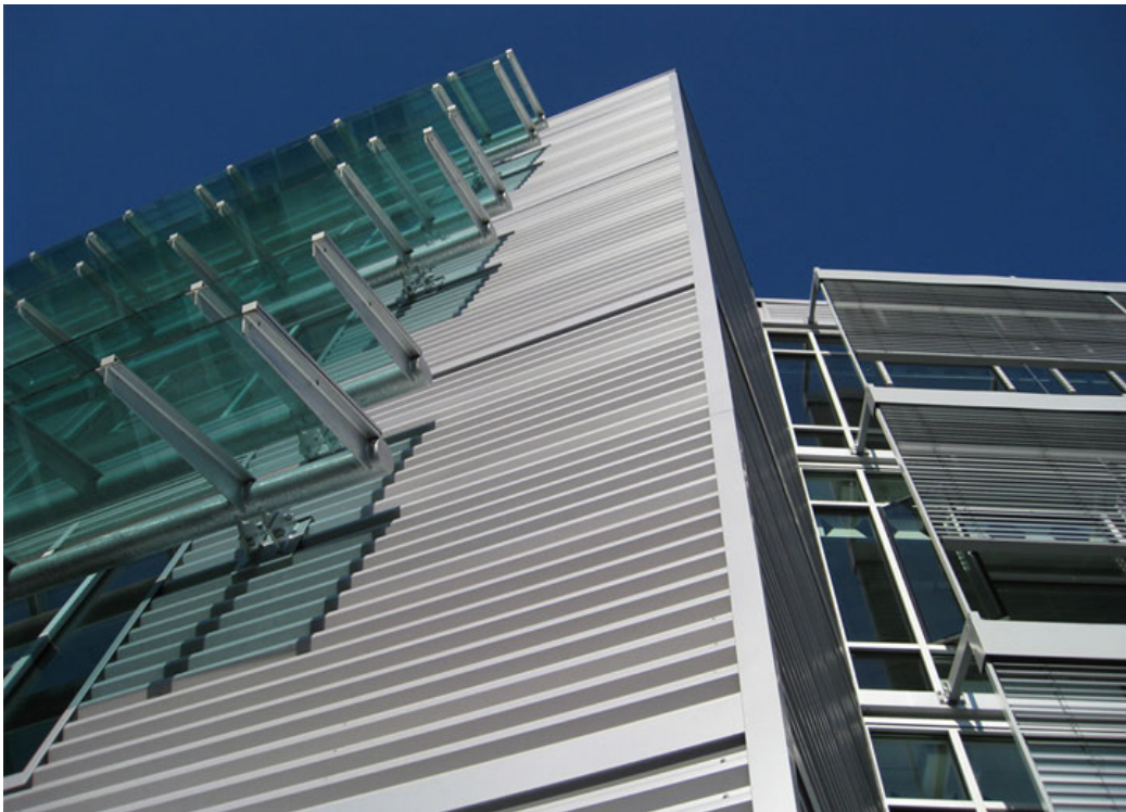
Figure 28.0: Glass sunshades (left) and operable blinds (right)
