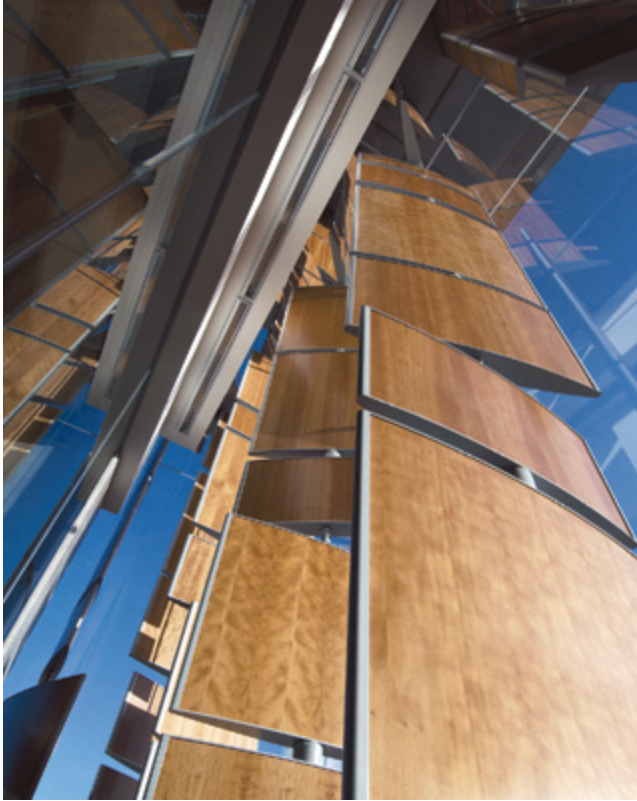
Figure 17.0: wooden louvers as double-skin façade
