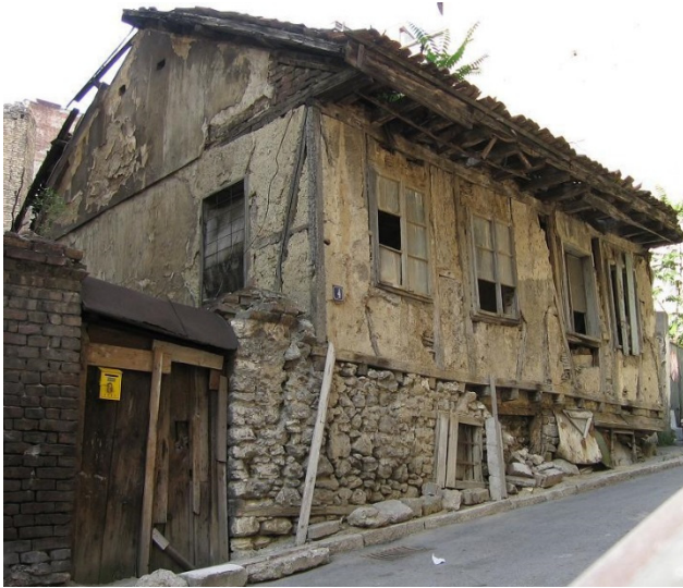
Figure 7. Example of straw cavity infill home in Serbia, house of Mr. Dimitrije Mirković, 1850.
