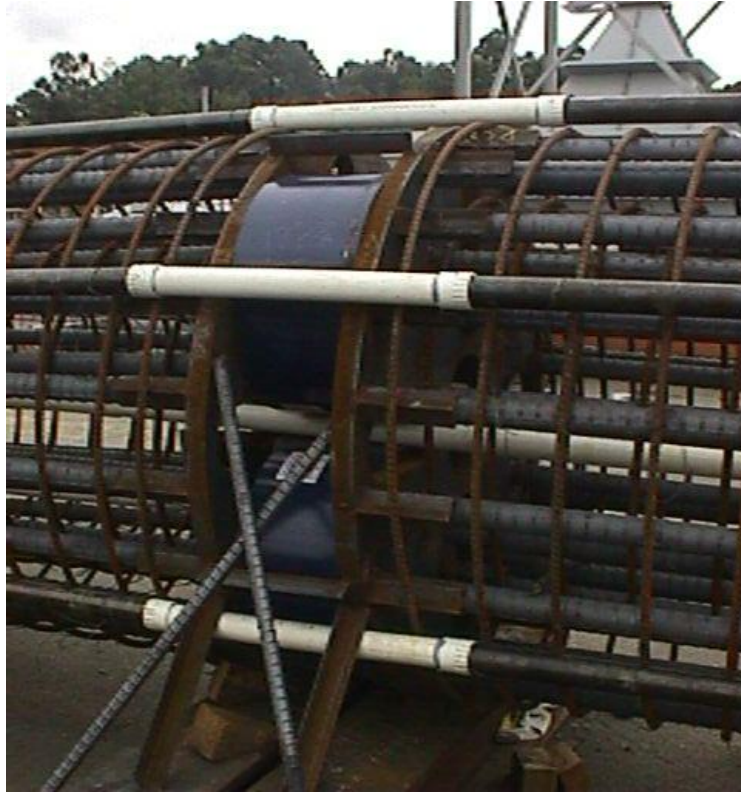
Figure 4-2: O-cell Installation in a Drilled Shaft (Caltrans, 1998)
