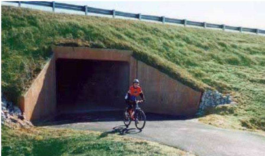
Figure 2-5. Underpass Pedestrian Crossing Below a Highway (Turner et al., 2006)
