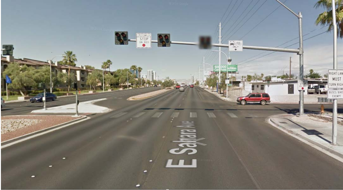
Figure 3-8. View of PHB System (Facing West on Sahara Ave., Google Map)
