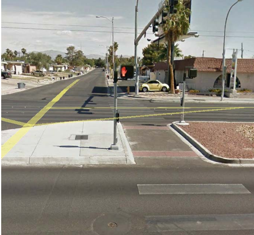
Figure 3-10. View of PHB System (Facing North on S. 15 th St., Google Map)
