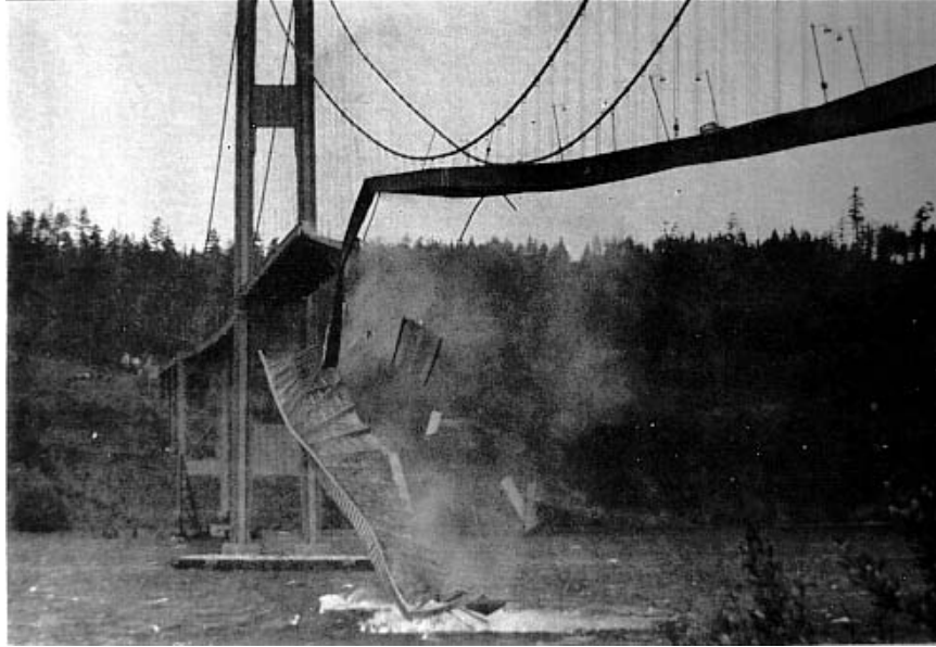
Figure 1.4. Collapse of the first Tacoma Narrows suspension bridge [Wikipedia (b)]
