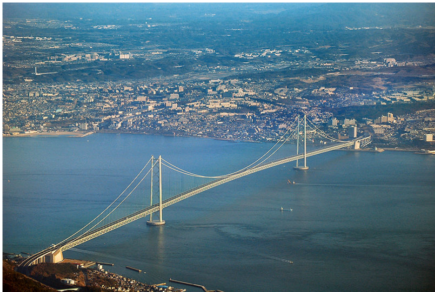
Figure 1.2. The Akashi Kaikyo suspension bridge [Wikipedia (a)]
