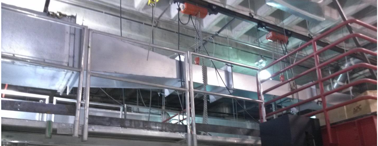
Figure 5.3: 12x18 Duct Test Setup
