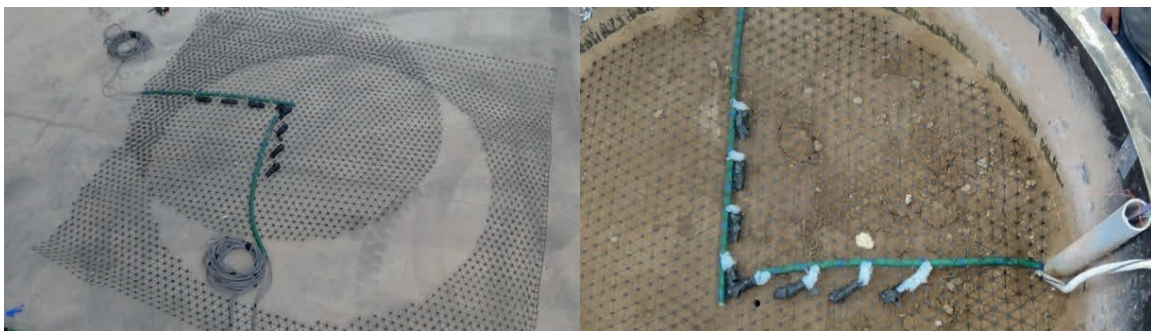
Figure 3.9: Geogrid installation
