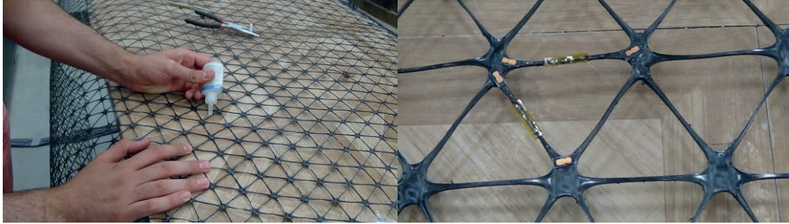
(a) (b) Figure 3.6: Foil strain gauge installation
