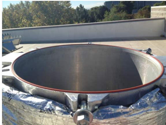
Figure 17: Autoclave with O-ring
