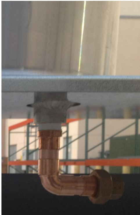
Figure 22: Copper piping that attaches to autoclave
