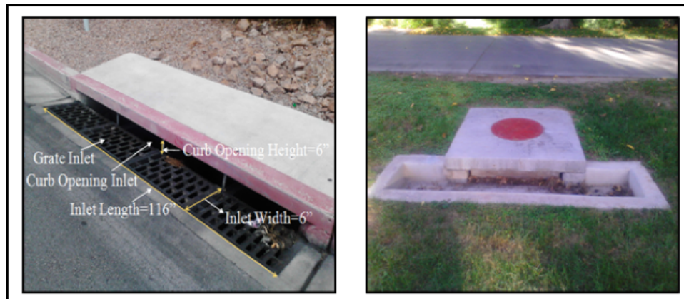
Figure 6. Storm drain inlet in Blacklot study site (on the left) and East Mall study site (on the right).
