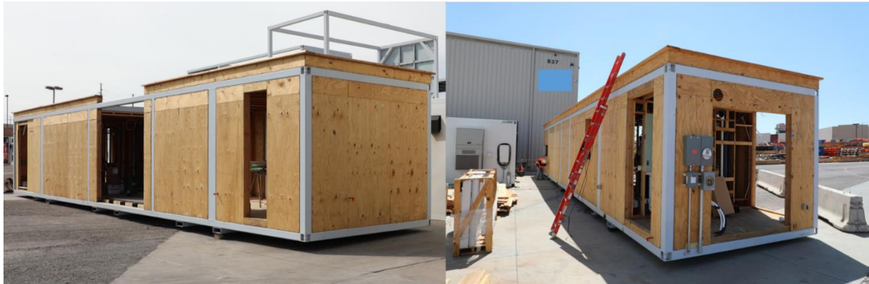
Figure 1. UNLV's Solar Decathlon 2020 project in progress
