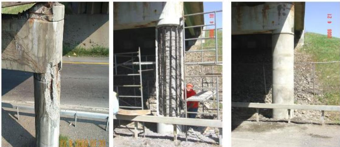
**Figure 10.** (Left) Corrosion Damage, (Center) Removal of Concrete and Repair Reinforcement, and (Right) Replace Concrete (NYDOT, 2008)
