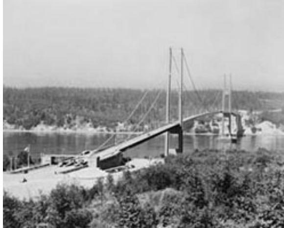
Figure 1.1. Tacoma Narrows Bridge before collapse. (WSDOT photo).
