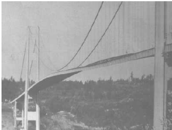
Figure 1.2. Tacoma Narrow Bridge very shortly before collapse, November 7, 1940. Note the combination of vertical and torsional deflection that eventually caused the structure to fail. (photo:www.ketchum.org)
