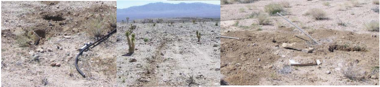
Figure 2.1 Vandalism and theft at the Morningstar mine.
