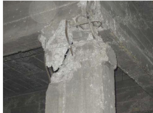
Sirinyurt apartment building
