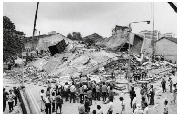
after collapse (Asiaone News, 2016)
