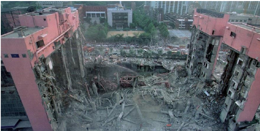
Figure 1.1 Collapse of Sampoong Department Store (Park, 2012).
