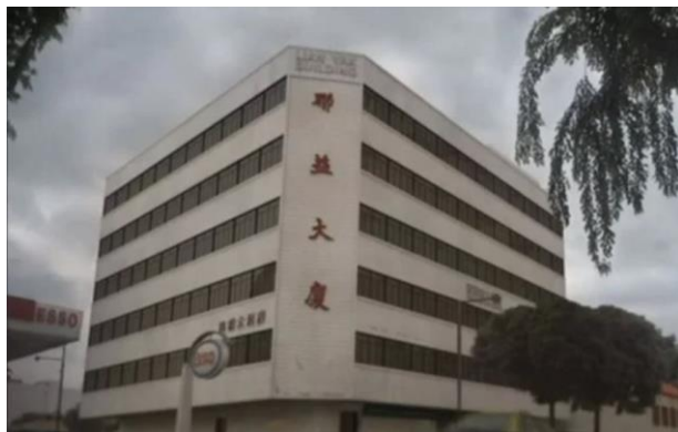
before collapse (MustShare News, 2016)
