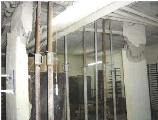
Altinbasak apartment building
