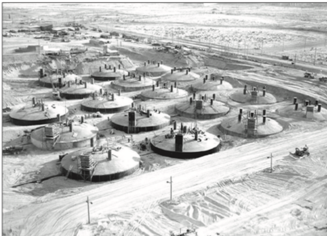
Figure 3: Hanford site tank farm 241-TX being backfilled [22].
